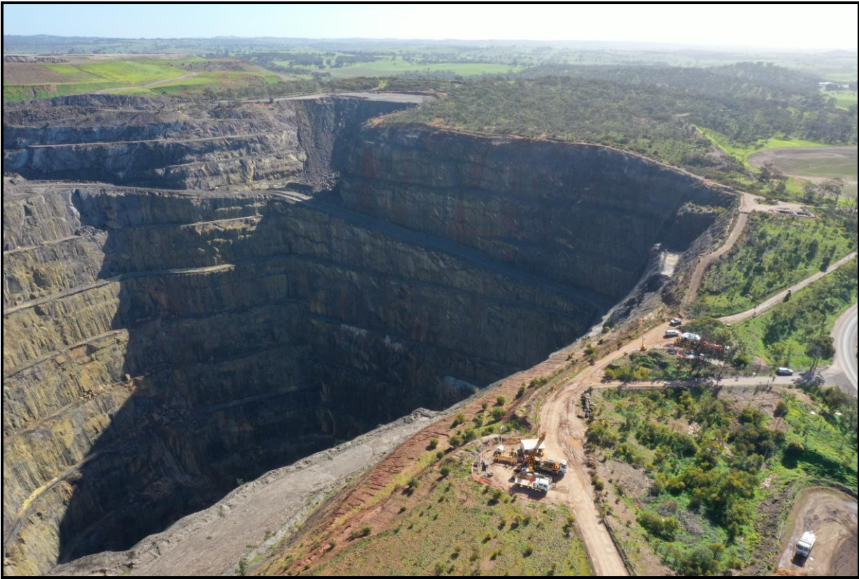
Figure 2 Location of Diamond Drilling sites – Aerial View looking nor-nor-west across the Giant open pit
