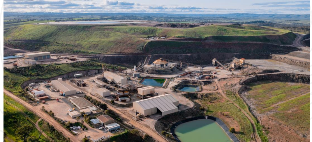
3.6MTPA PROCESSING PLANT
