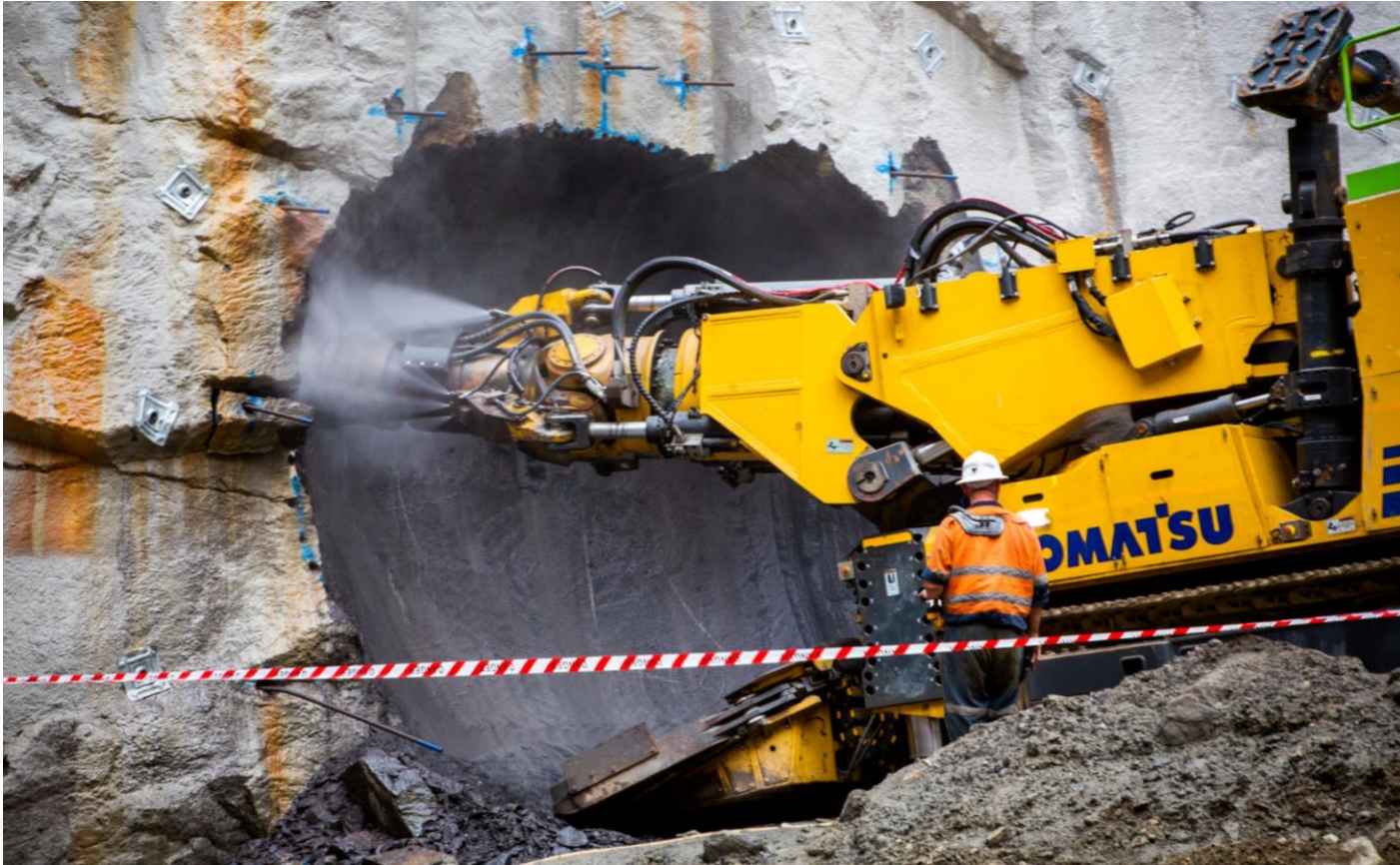
COMMENCEMENT OF THE PORTAL FOR UNDERGROUND DECLINE
