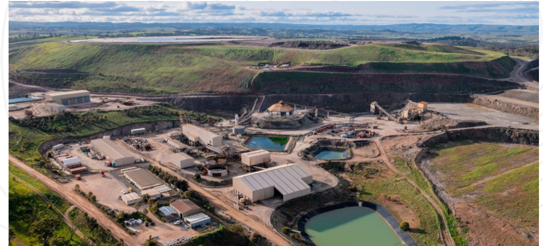
3.6MTPA PROCESSING PLANT
