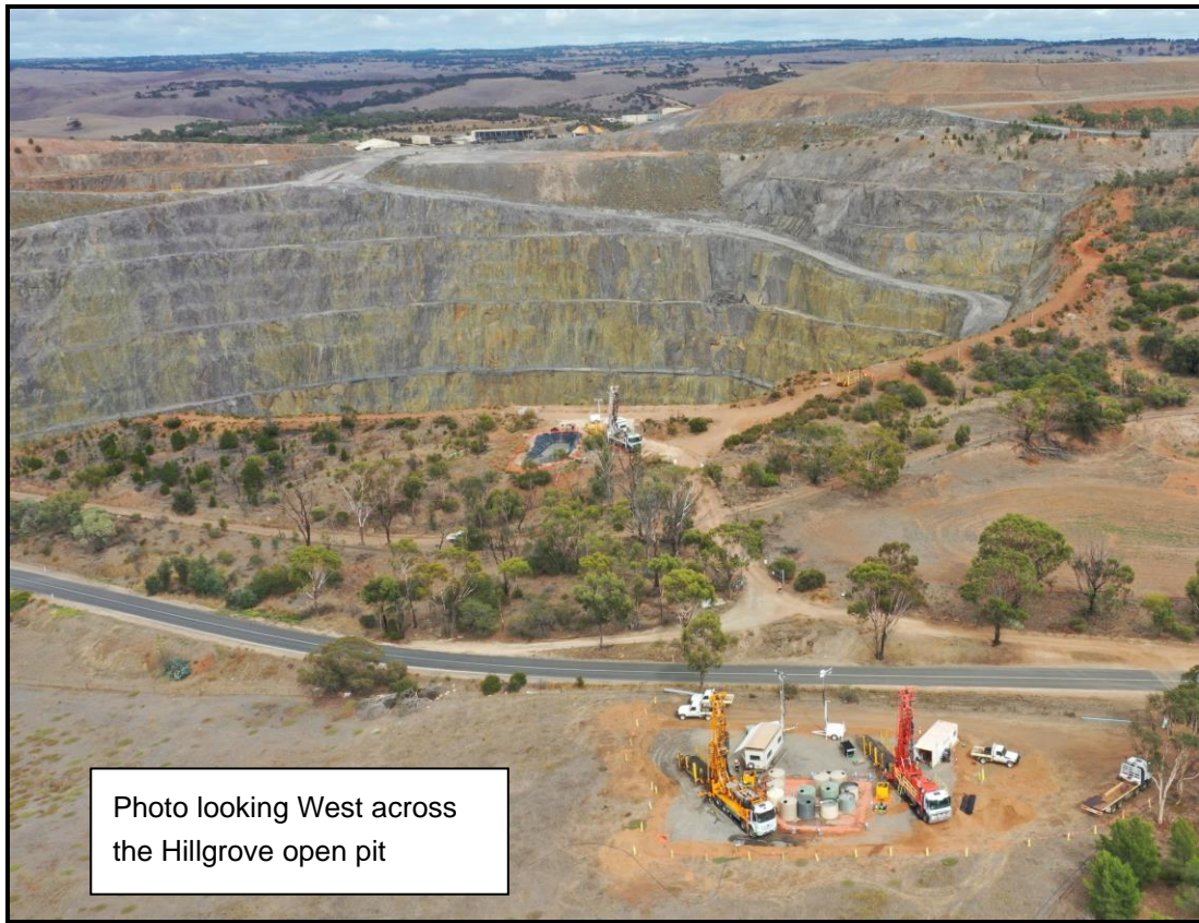
Figure 2 Location of Diamond Drilling – Aerial View
