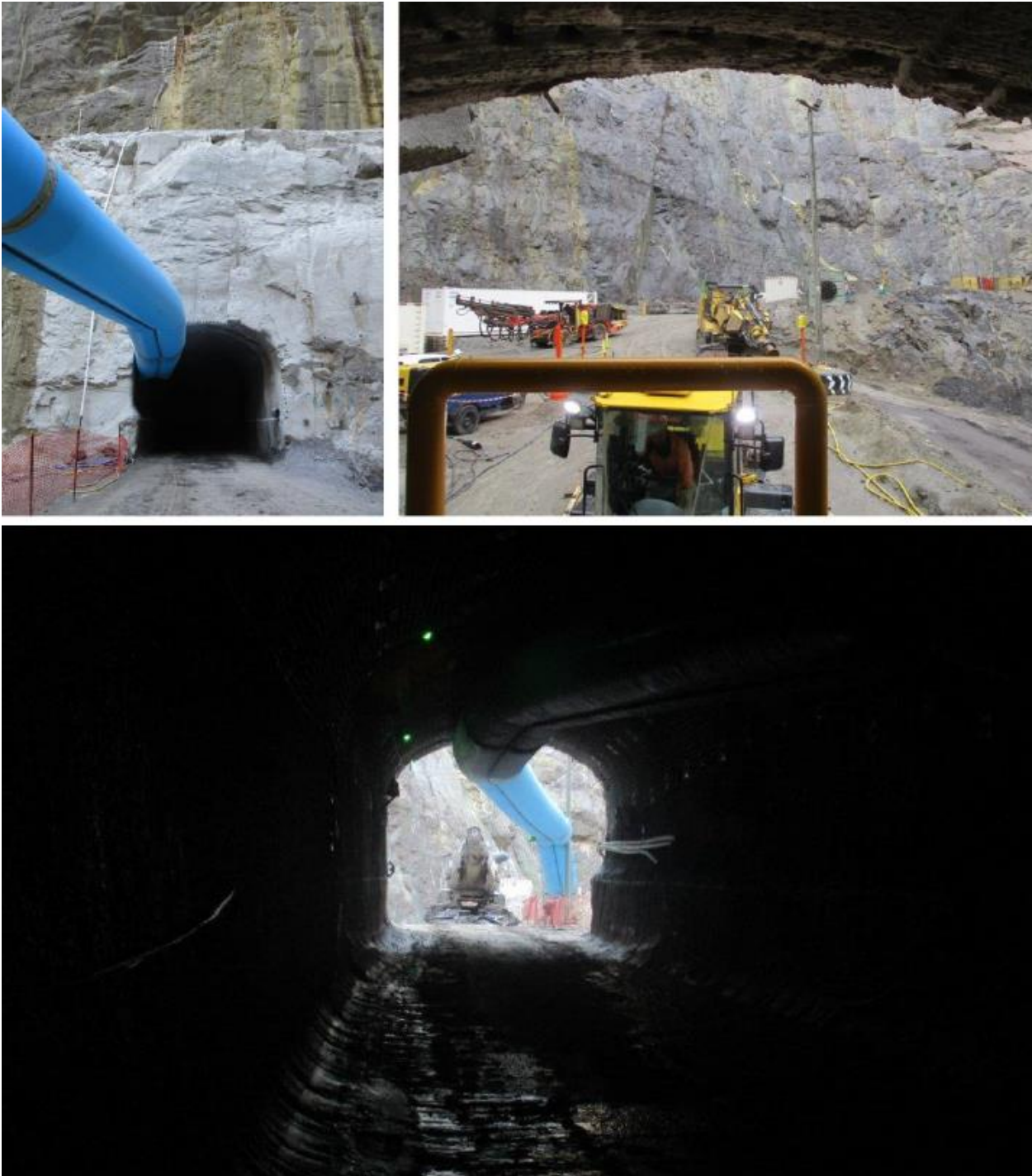
Figure 2 Portal complete (LHS) and view looking out from inside the portal (RHS) and view from within the decline (lower image)
