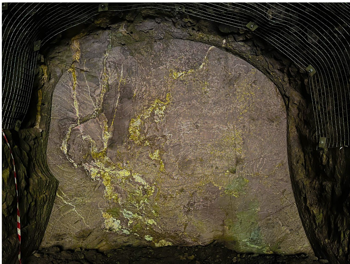
Figure 2 Scan of the copper mineralisation as exposed in the UG ventilation drive
