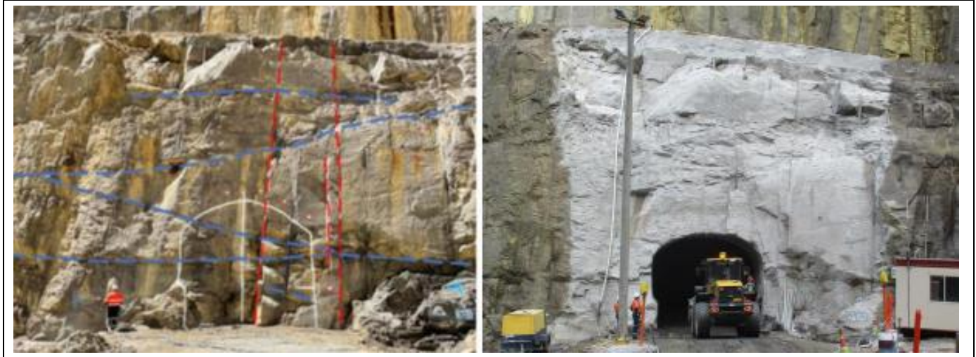
Figure 10: Mapping of the exploration decline portal face (left) and the established portal (right)
